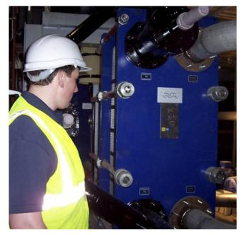
Two plate heat exchangers from Alfa Laval maintain the internal temperature in the produce depot at a constant  $+2^{\circ}C$ .
